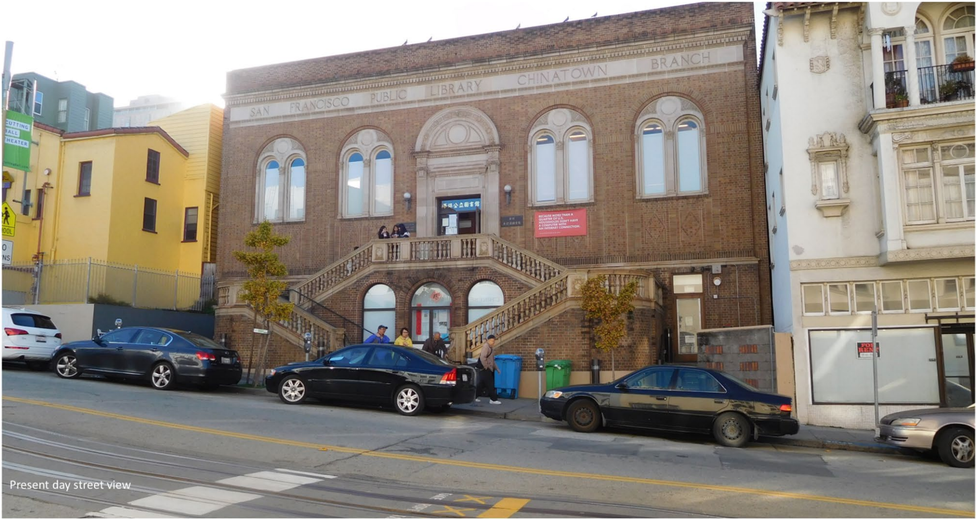
Chinatown Branch Library Renovation | Bureau of Architecture
