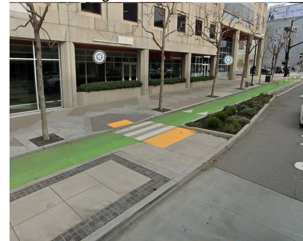
New Parking & Island Protected Bike Lane
