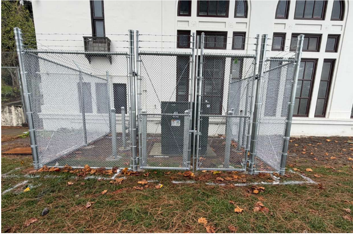
Pumping Station No.2 Electrical equipment installation
