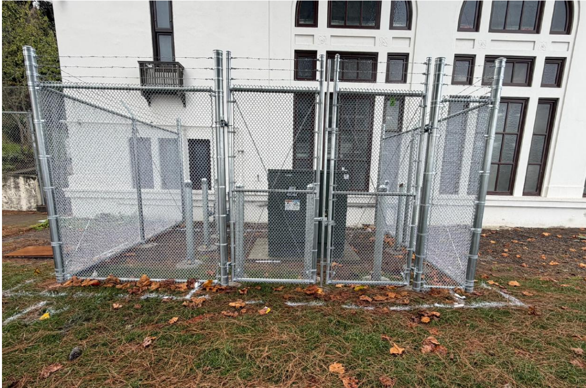
Pumping Station No.2 Electrical equipment installation
