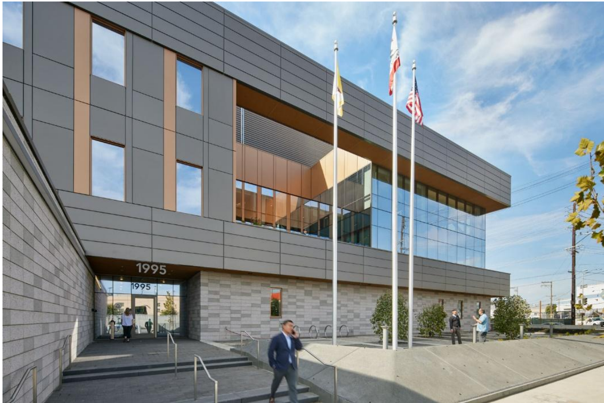
Photos by Bruce Damonte
