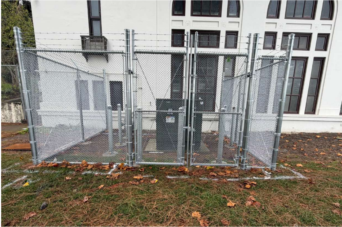
Pumping Station No.2 Electrical equipment installation
