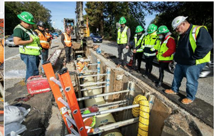
19th Avenue – Installation of the 36-inch pipeline
