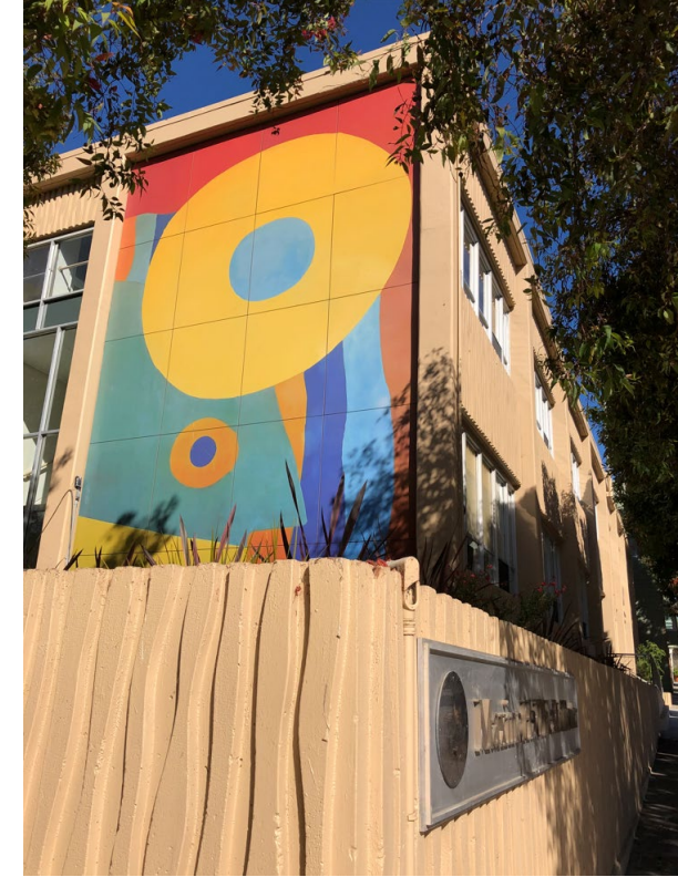
View of southeast corner showing new shear wall.
