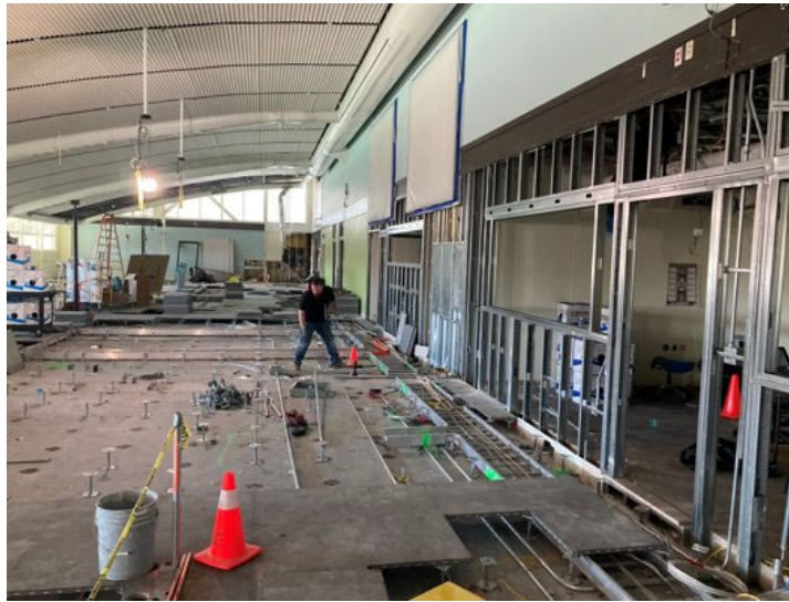
911 Call Center construction at the City's Emergency Operations Center
