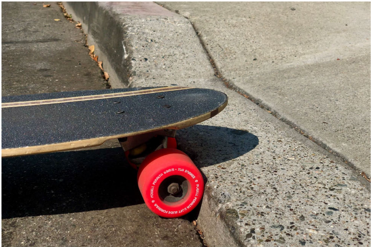
[Item 4]: An example of a driveway curb lip on Shotwell Blvd which exceeds the specified one-inch height
