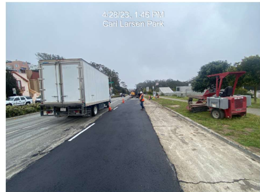
Paving on 19th Ave after the PEFWS 36-inch pipe installation
