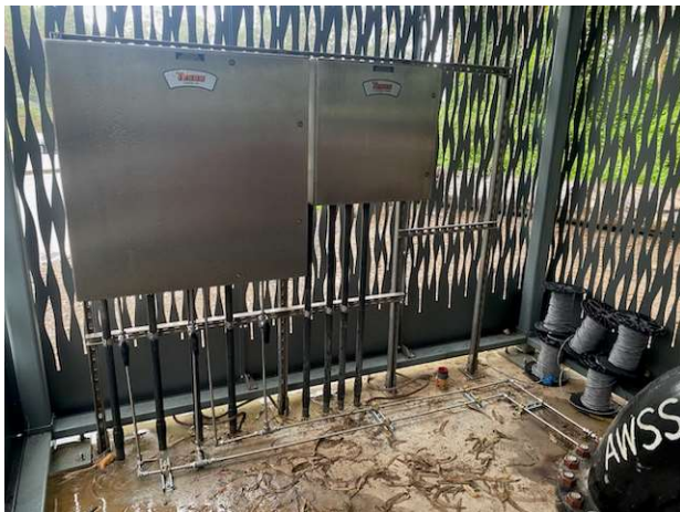
Clarendon Supply Site – SCADA Installation
