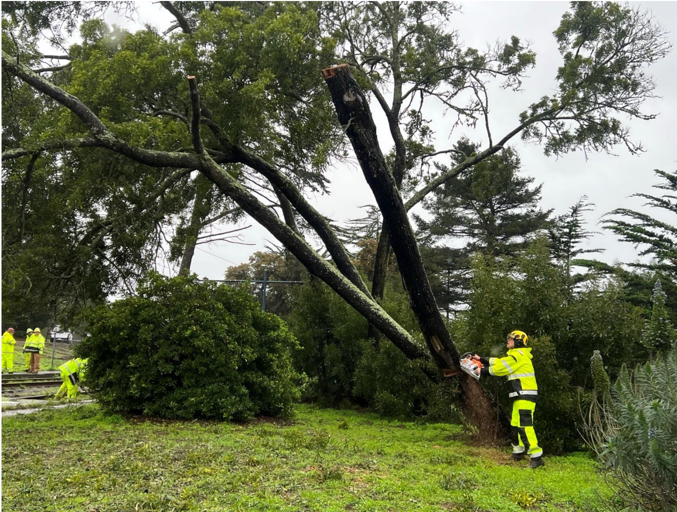
Tree removal at Junipero Serra and Sloat streets.
