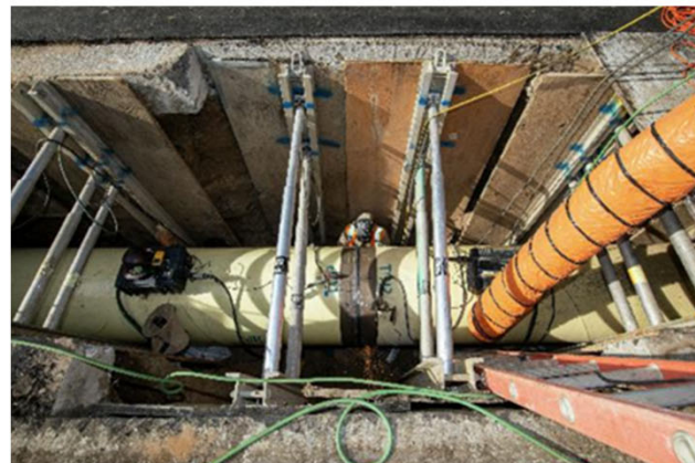
19th Avenue – Installation of the 36-inch pipeline
