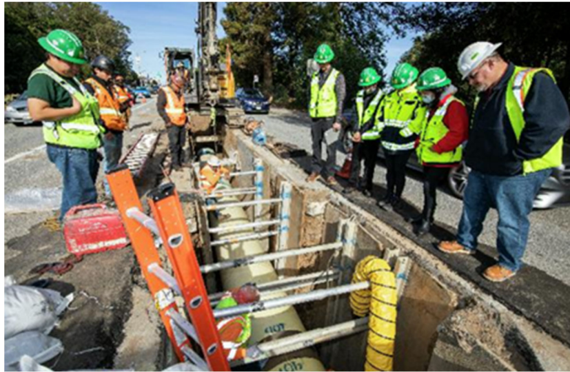
19th Avenue – Installation of the 36-inch pipeline, EFWS 2020
