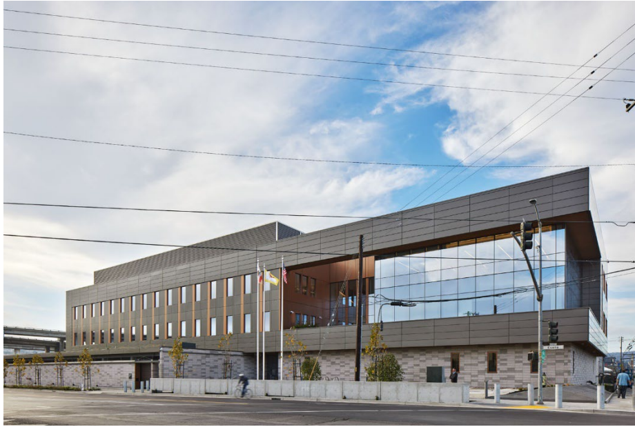
North façade at Evans Avenue intersection with Toland Street
