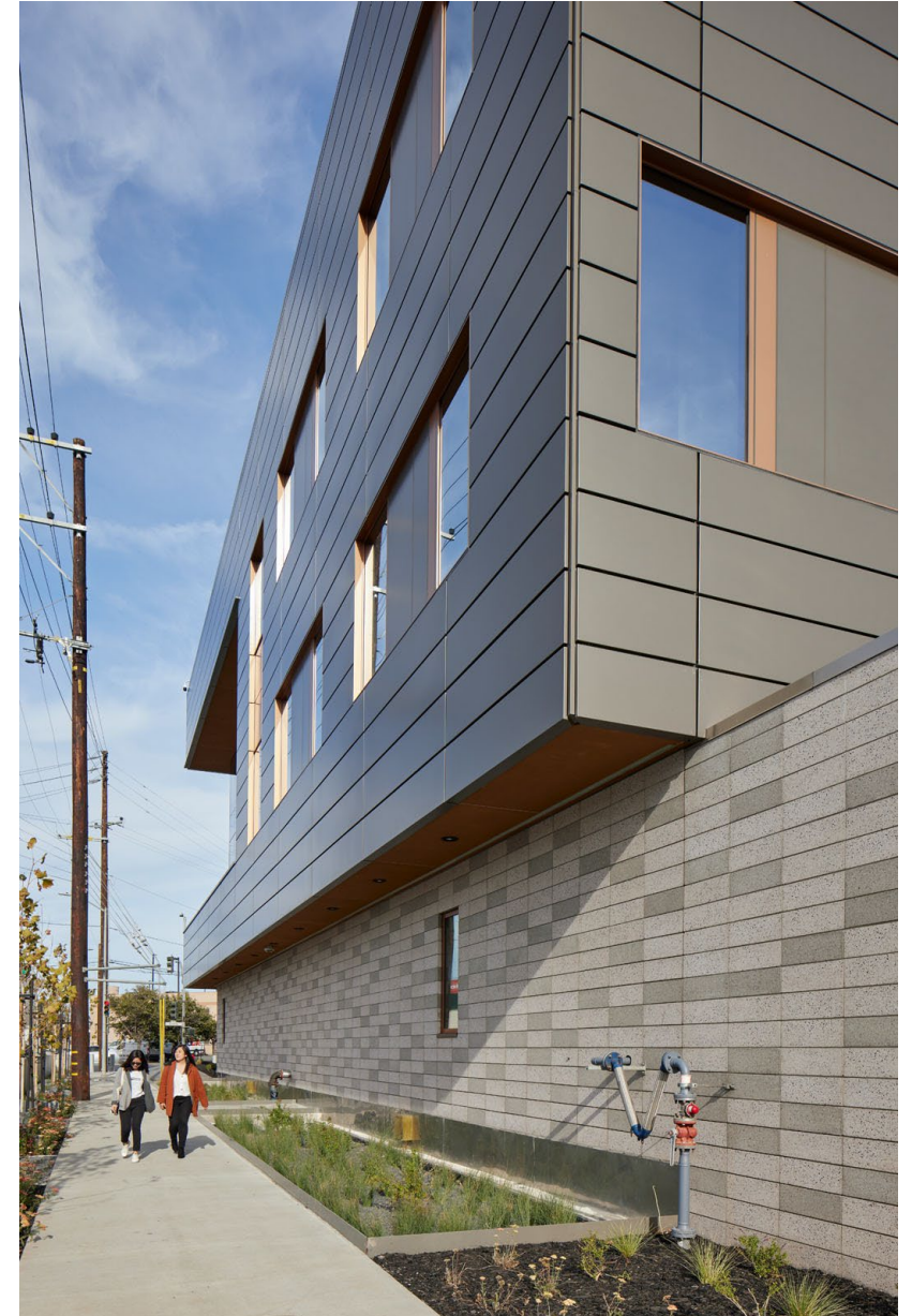
North façade at Toland Street
