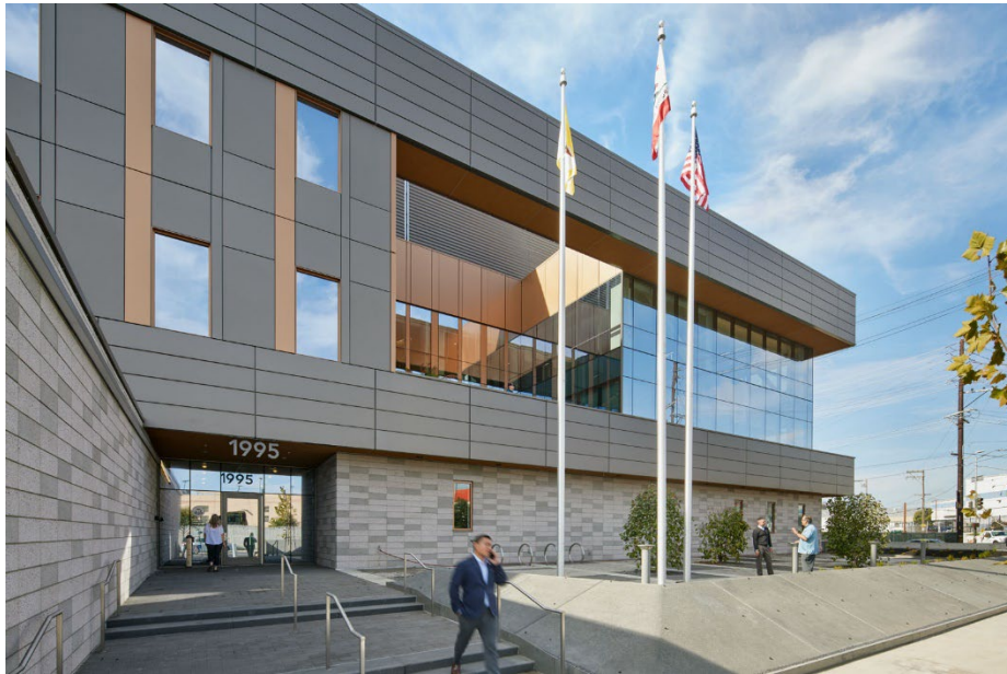
Main entry and plaza at Evans Avenue
