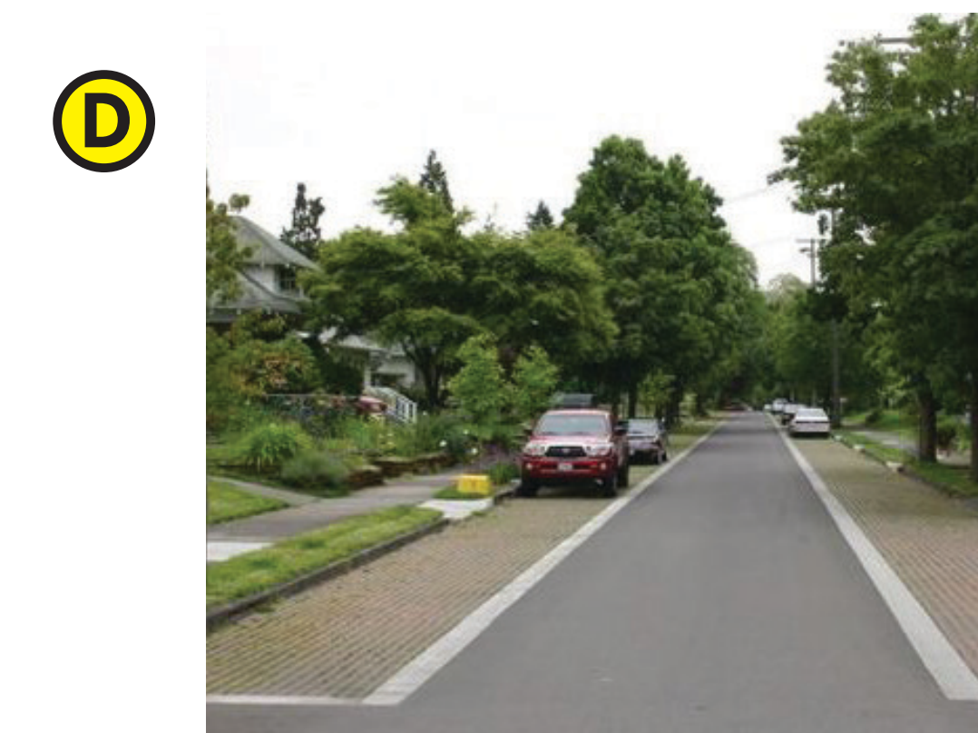
D PERMEABLE PARKING STRIP Permeable pavers located along the parking strip allow for stormwater infiltration
