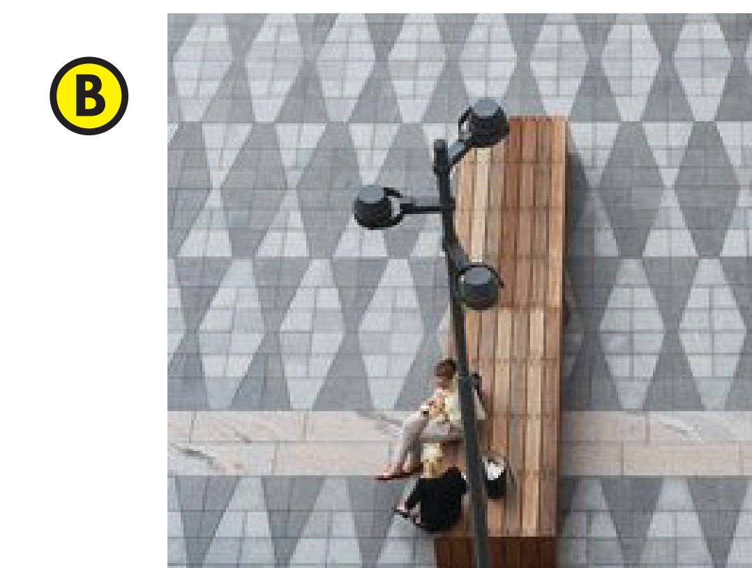
B PERMEABLE PAVING
