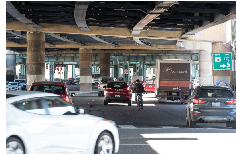
Existing condition from 13 th St/Duboce St/Mission St intersection looking east
