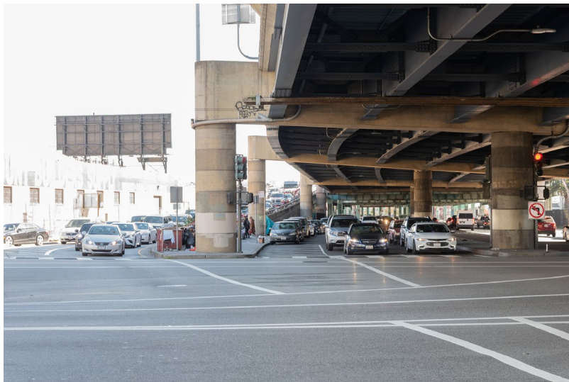
Existing condition from 13 th St/Duboce St/Mission St intersection looking east
