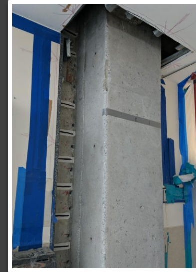
BEFORE AND AFTER FRP INSTALLATION
