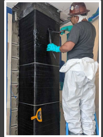
BEFORE AND AFTER FRP INSTALLATION
