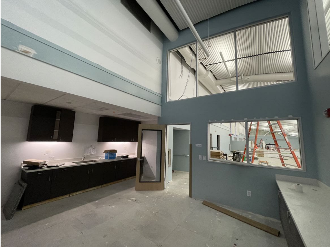
Break Room— During Construction
