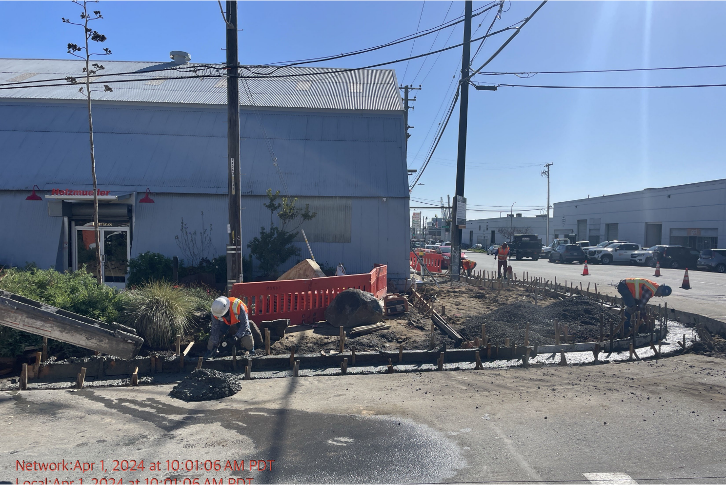
25th & Minnesota NE Corner New sidewalk, corner bulb-out, curb ramps
