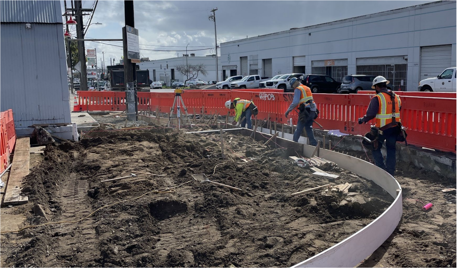
25th & Minnesota NE Corner New sidewalk, corner bulb-out, curb ramps
