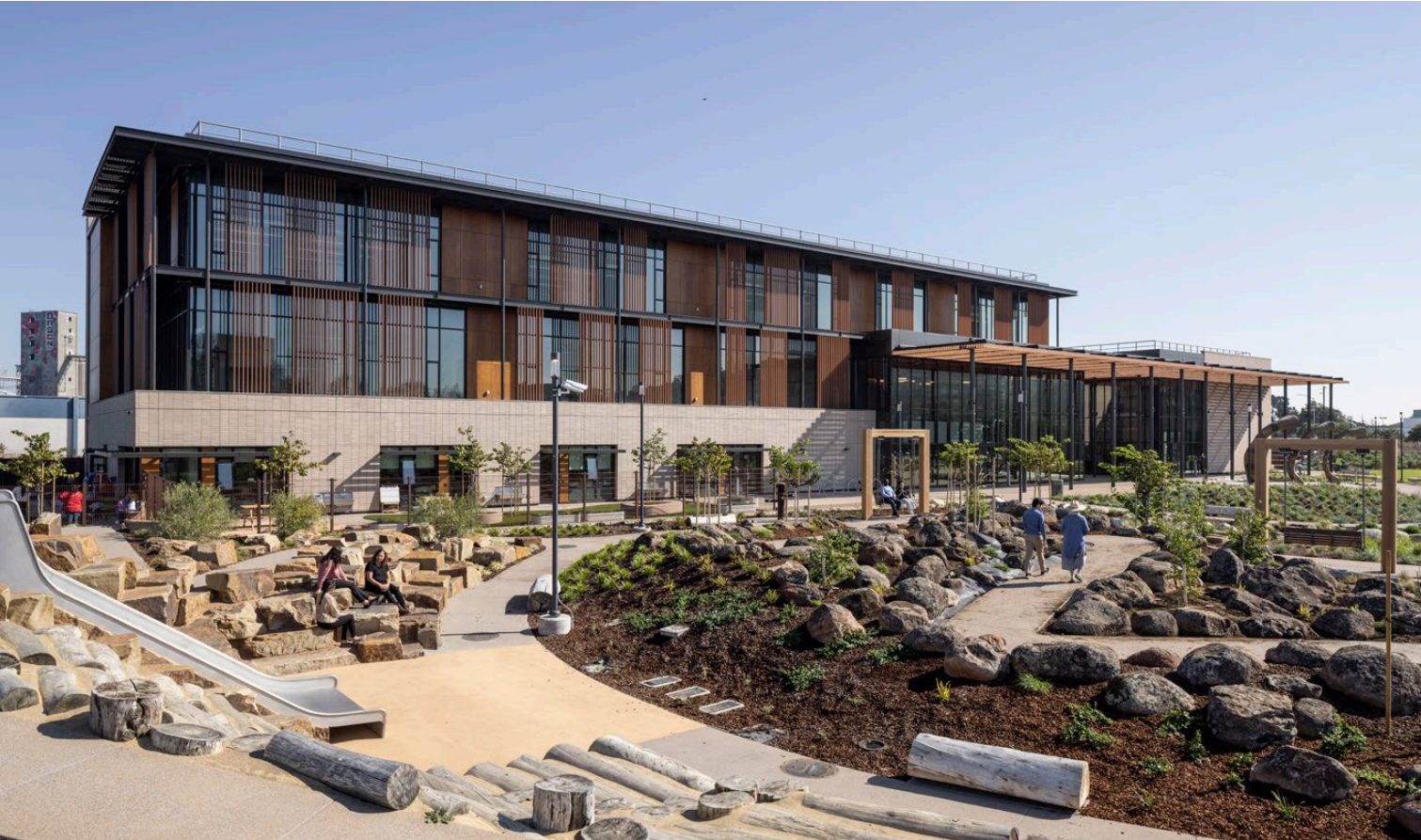
The Southeast Community Center is a LEED Gold-certified, all-electric facility with rooftop solar panels.
