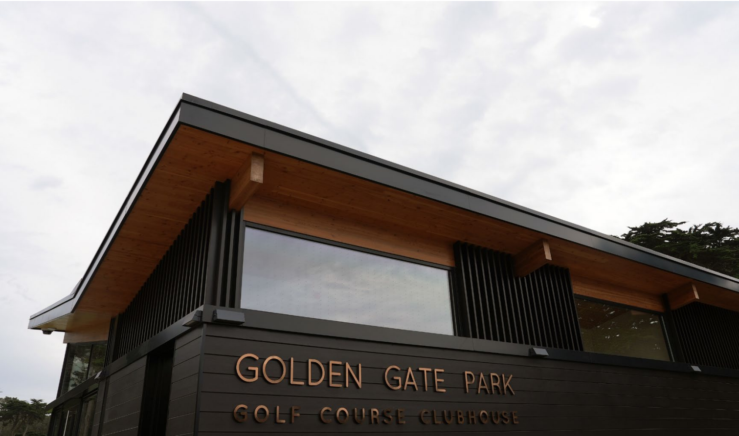
The Golden Gate Park Golf Course Clubhouse's design and materials incorporate smart green-building practices, such as mass timber.
