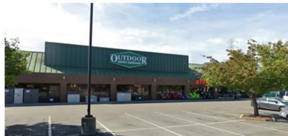
⑧ OSH RETAIL BUILDING AND PARKING LOT
