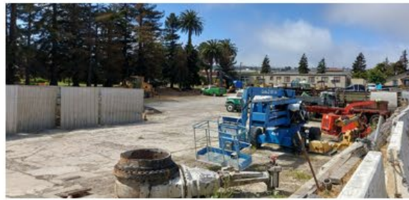
② SITE PIT FROM REMAINING OLD BUILDING
