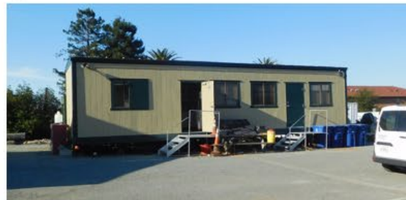
⑥ TEMPORARY TRAILERS TO HOUSE GROWING STAFFING NEEDS
