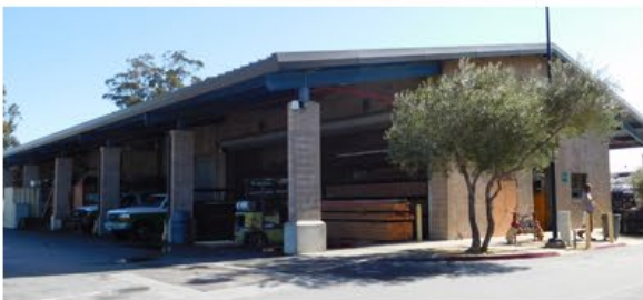
⑦ NORTH SHOP BUILDING
