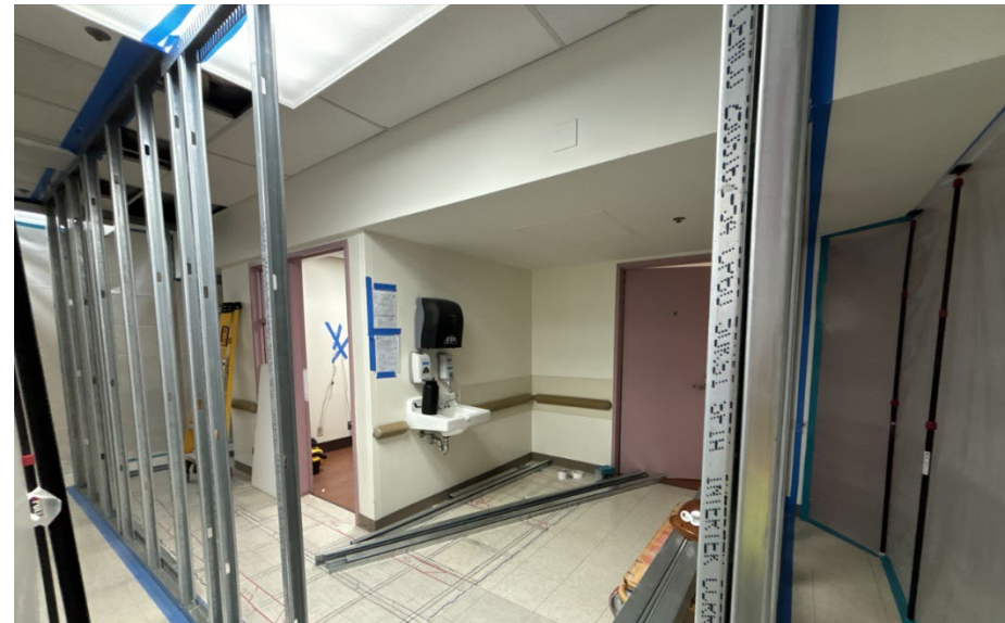
3C Accessible Restroom – Temp Construction Barrier Installation
