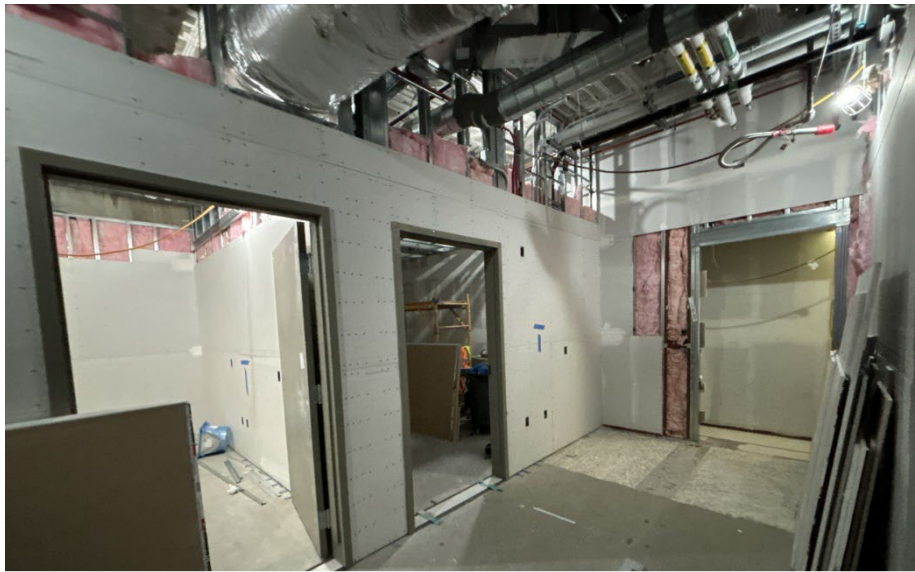
Urology – Partition Wall and HVAC Installation
