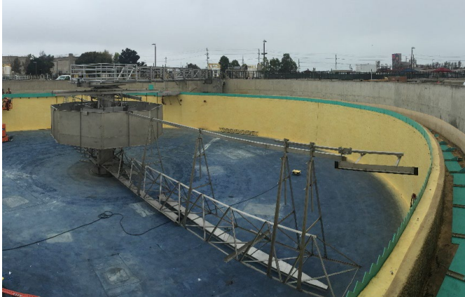
Southeast Plant Primary & Secondary Clarifier Upgrade
