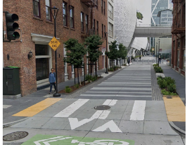
New Raised Crossings and Roadway
