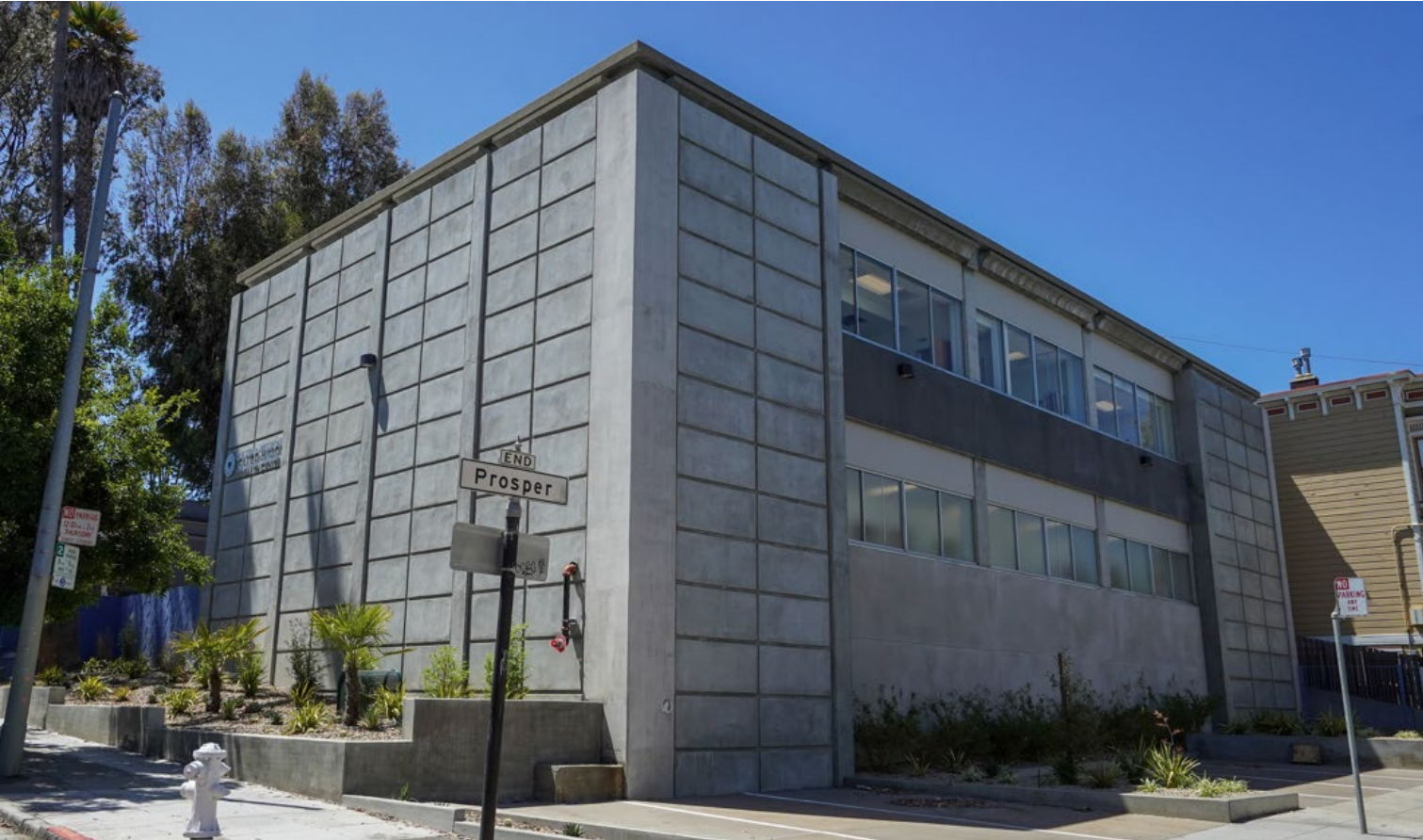
Front view along Prosper Street.
