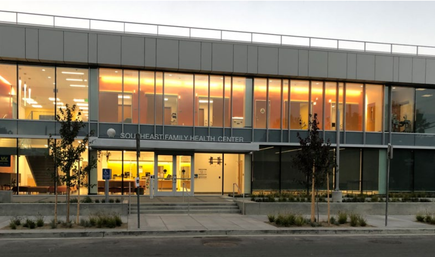
Front view along Keith Street.
