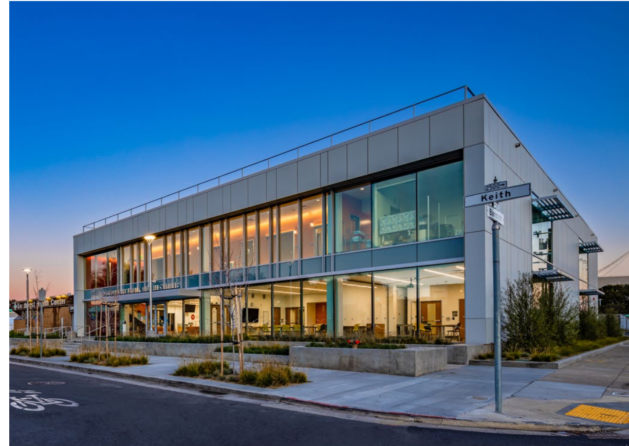
View of southwest corner of new facility.
