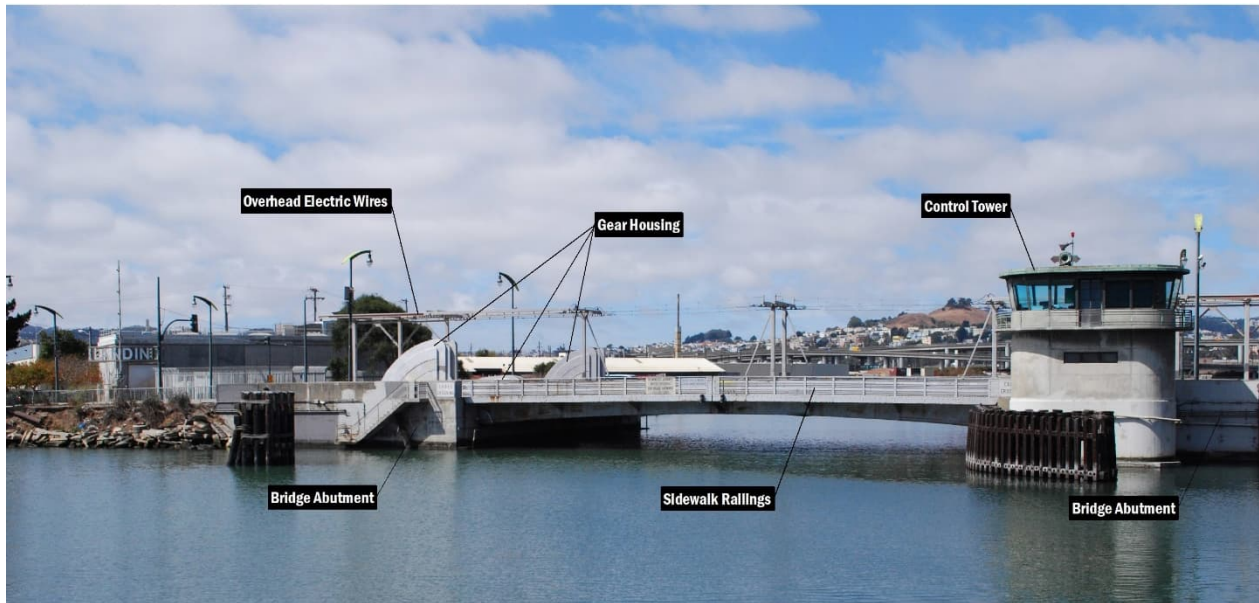
Figure 2 Islais Creek Bridge East Elevation
