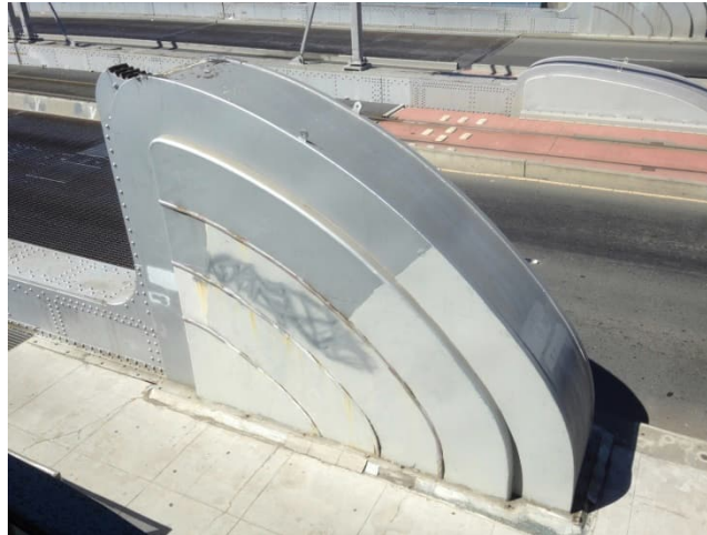
Figure 3 Quarter-Circle Gear Housing showing Art Moderne Style Applied to Bridge
