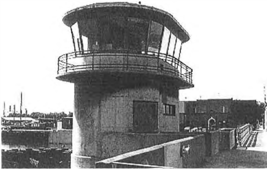
Detail of the control tower. May 2004.
