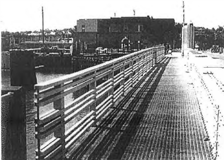
Detail of sidewalk (open, metal grate) and railing. May 2004.
