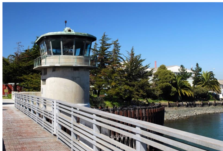
Figure 4 Control Tower and Sidewalk Railing showing Art Moderne Style Applied to Bridge
