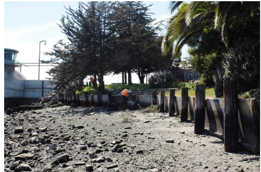
Photo 8: Northeastern side of bridge, western aspect (mudflat during low tide).
