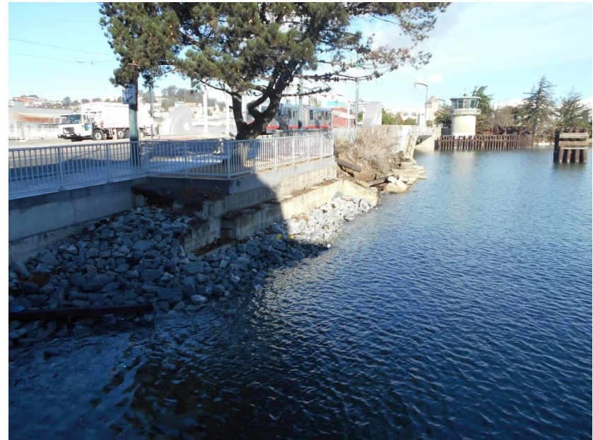
Photo 12: Southeastern side of bridge during high tide, northern aspect.
