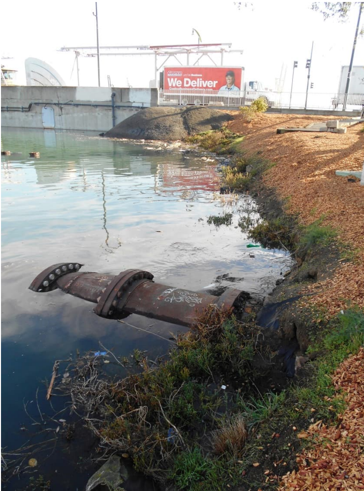
Photo 9: Southwestern side of bridge during high tide, northeastern aspect.
