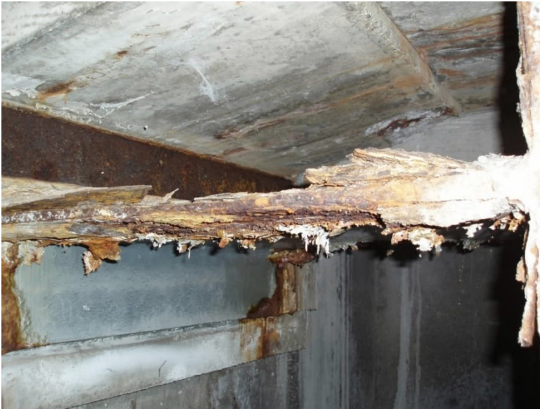
Photos 1 and 2: Corrosion Under the Bridge Deck Corrosion and Concrete Cracks in Bridge Deck
