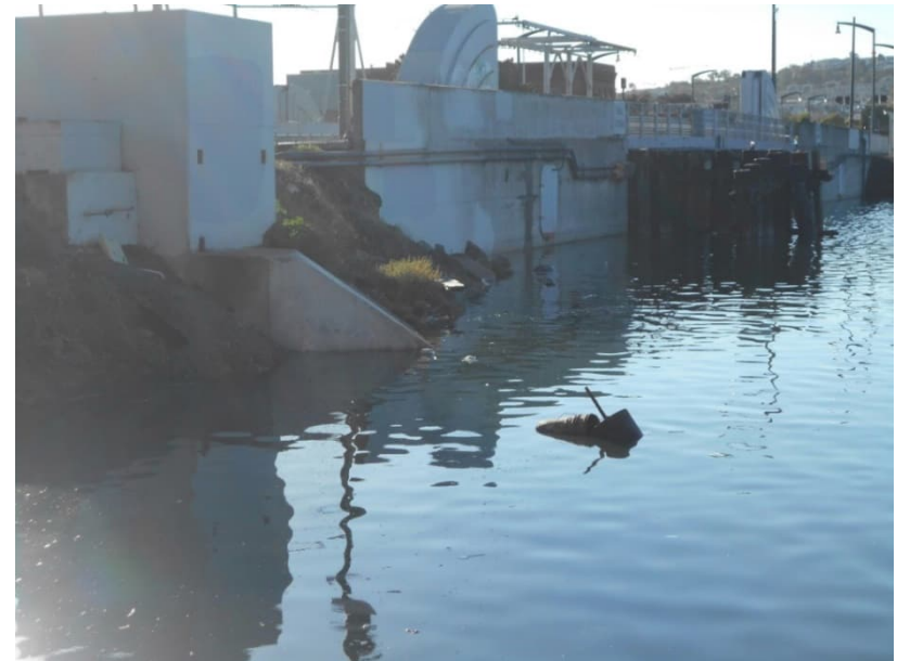
Photo 14: Northwestern side of bridge, southeastern aspect.
