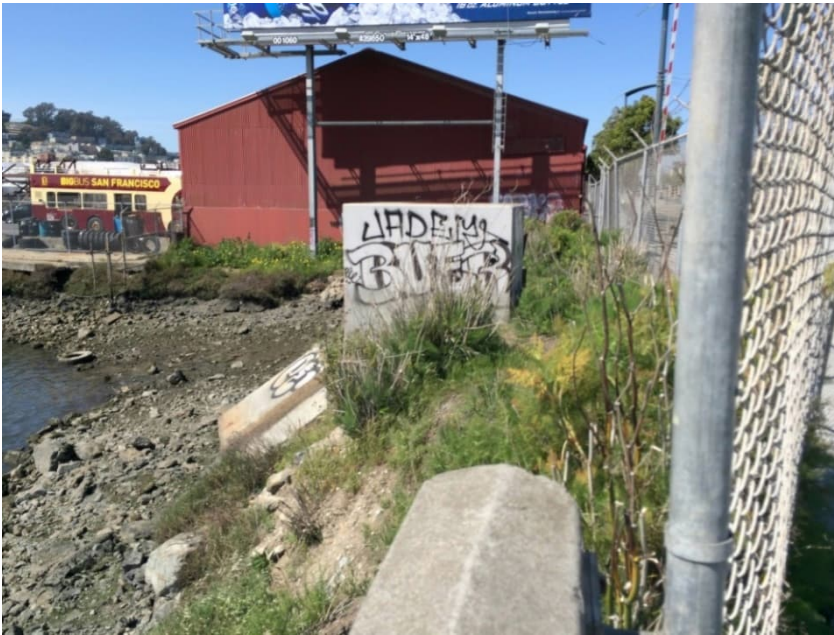
Photo 13: Northwestern side of bridge during low tide, northern aspect.
