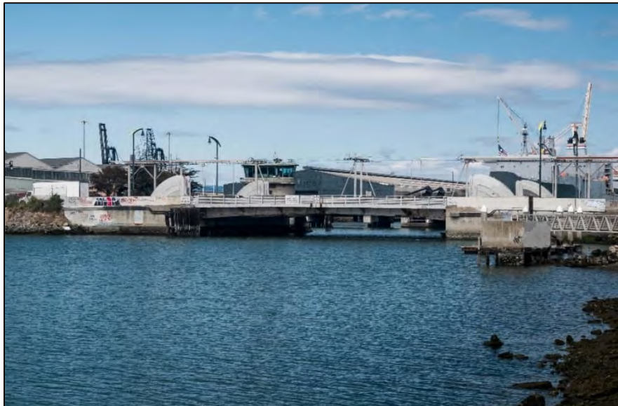
Photograph 2: Islais Creek Bridge, facing northeast
