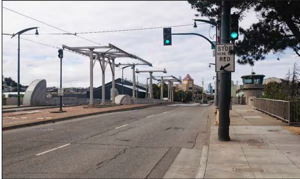
Photograph 7: Catenary poles for light rail trains, modern light fixtures and traffic gates, and replacement control gates, facing northwest
