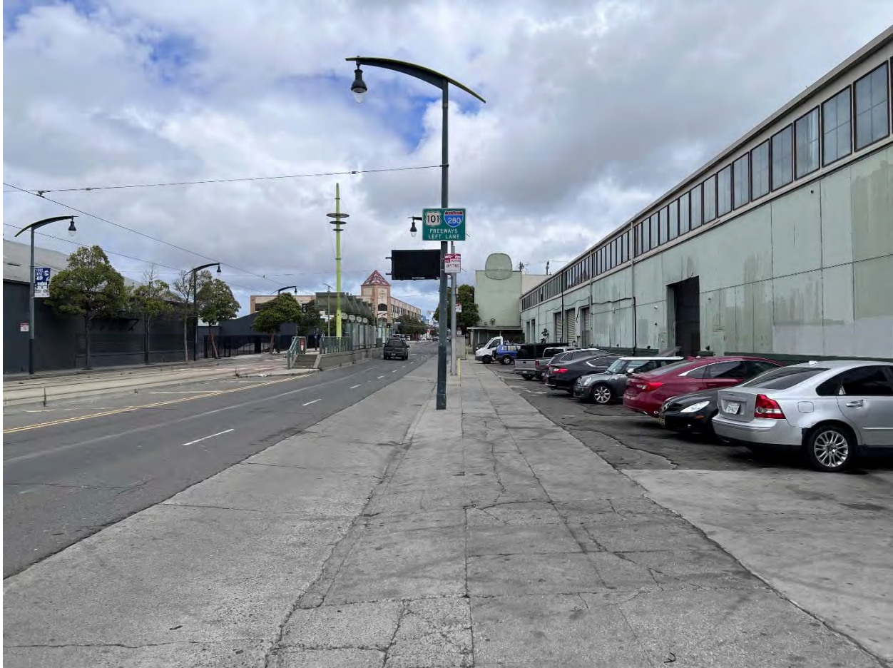
Photograph 11: View of southern boundary of Central Waterfront / Potrero Point Historic District from north side of Islais Creek Bridge as viewed along Third Street, view facing north, July 6, 2022.
