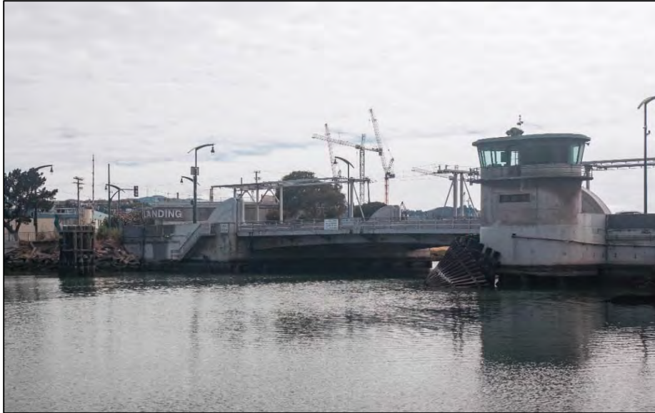
Photograph 1: Islais Creek Bridge with control tower at northeast corner, facing southwest
