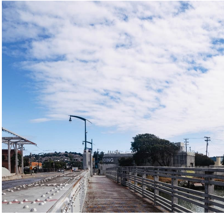
Figure 7: View from Islais Creek Bridge facing South Photo Date May 28, 2022.
