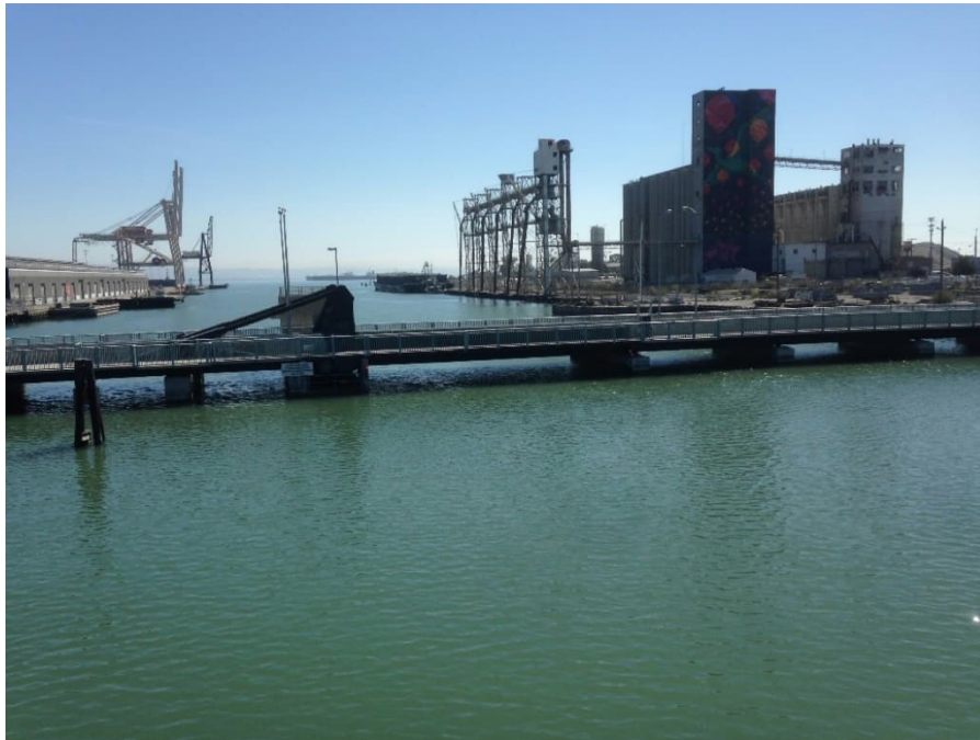
Figure 4: View from Islais Creek Bridge facing East Photo Date August 27, 2015.
