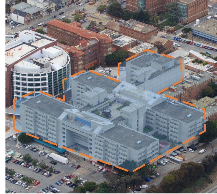
Aerial View of ZSFG Building 5
