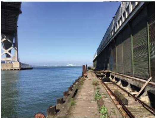
1 EXISTING FENDER SYSTEM AND ASPHALT TO BE REMOVED. EDGE BEAM RAIL TO REMAIN
