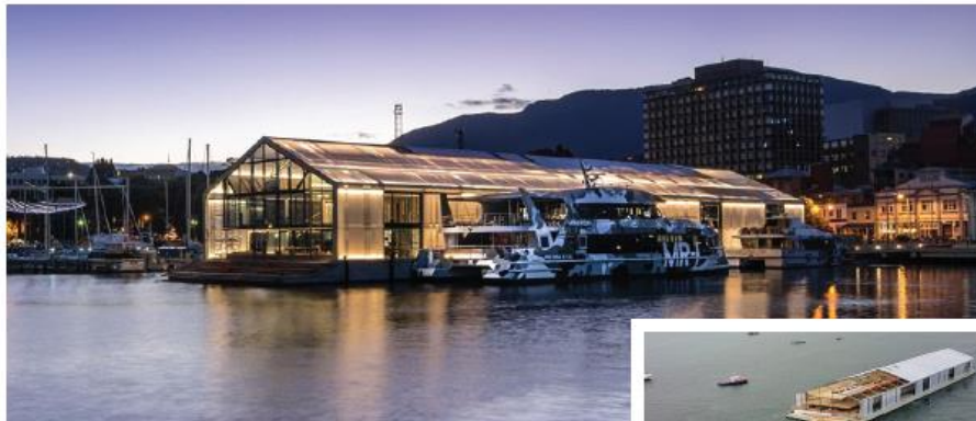
Brook St. Pier Ferry Terminal (Australia) Concrete Barge, Ferry Berth, mark and Restaurants.
