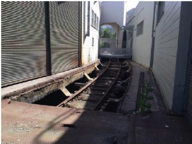
1 EXISTING FENDER SYSTEM AND ASPHALT TO BE REMOVED. EDGE BEAM RAIL TO REMAIN
