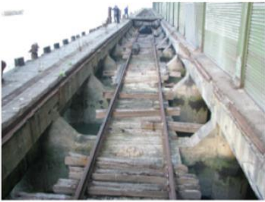
2 CURB ANGLES AND MISCELLANEOUS DEBRIS TO BE REMOVED EXISTING RAIL AND TIES TO BE PROTECTED IN-PLACE
