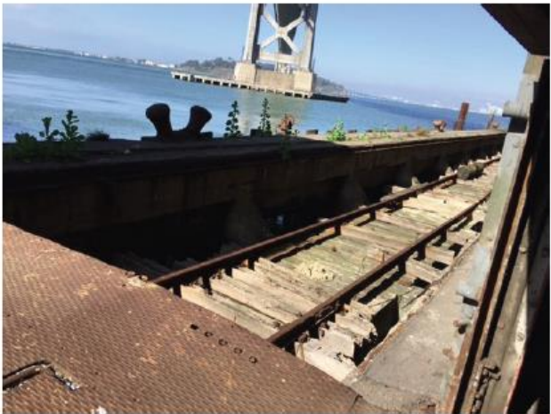
2 CURB ANGLES AND MISCELLANEOUS DEBRIS TO BE REMOVED EXISTING RAIL AND TIES TO BE PROTECTED IN-PLACE
