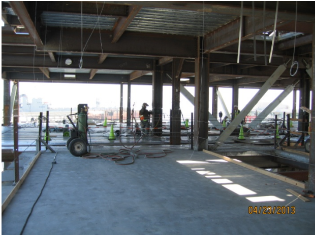
Finished concrete pour at 5 th Floor Staff Elevator Lobby
