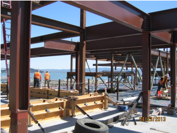
Steel framing for mechanical penthouse at Roof Level
