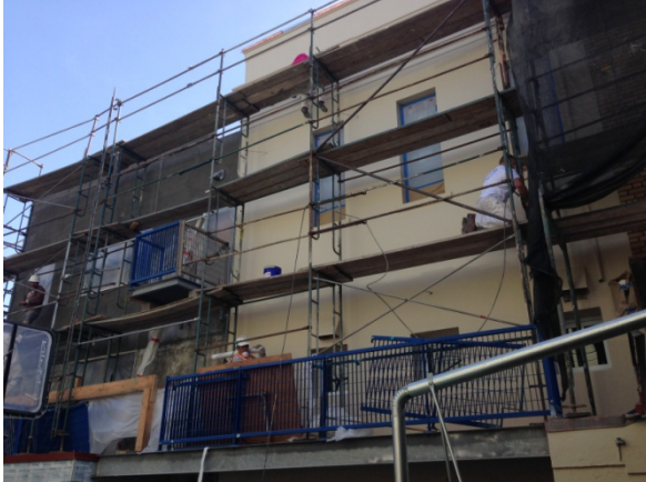
Scaffolding for Stucco
