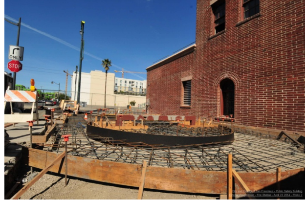
Preparation work for South Plaza
