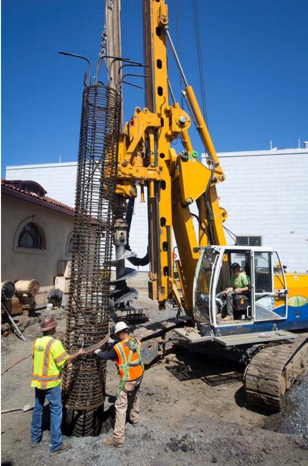
Drilled Pier Placement
