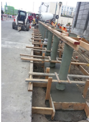
Bollard installation at 3 rd Street
