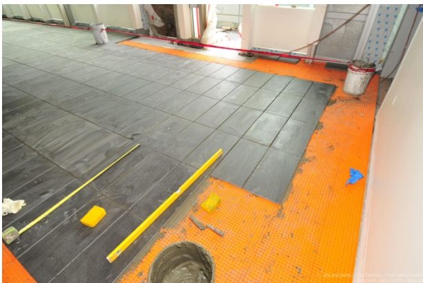
Tiling work at elevator lobby on Level 3
