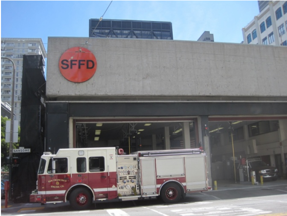
Fire Station 13 Concrete Sealer and Wall Panel Coating
