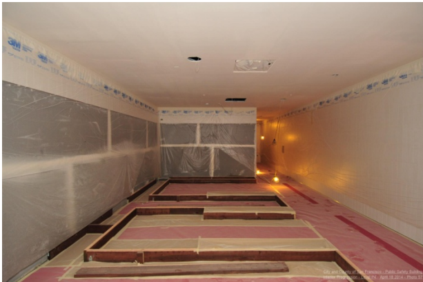
Preparation for locker installation at Level 3 Women's locker
