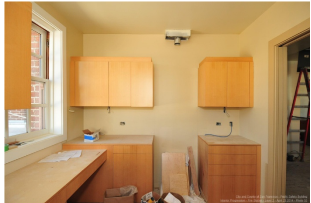
Cabinetry installation at FS30 - Arson Task Force
