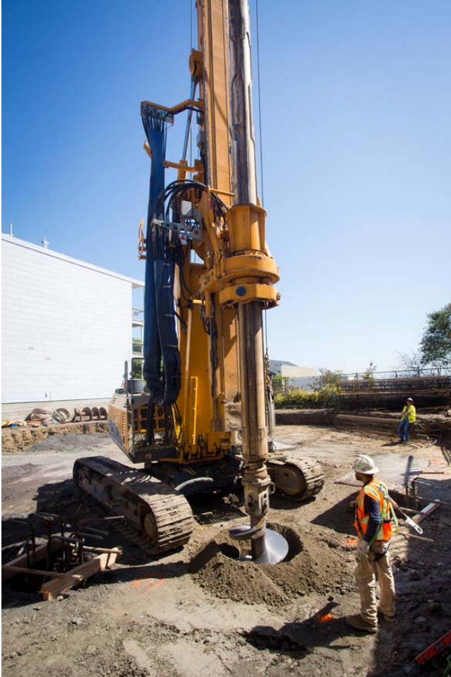
Drilled Pier Preparation
