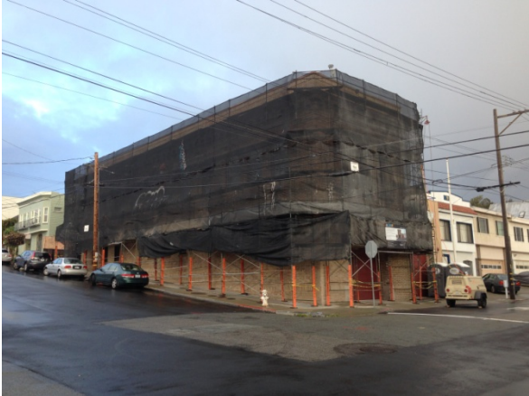
Brick Masonry at the Facade
