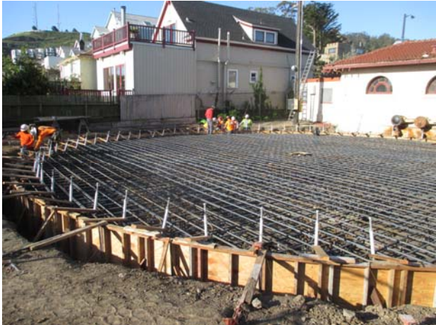
Foundation Slab Reinforcement
