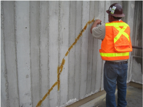
Station 26 Epoxy Injection
