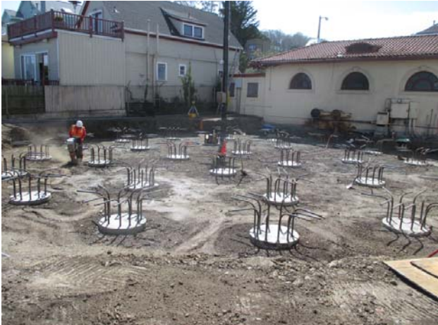
Multiple Drilled Piers
