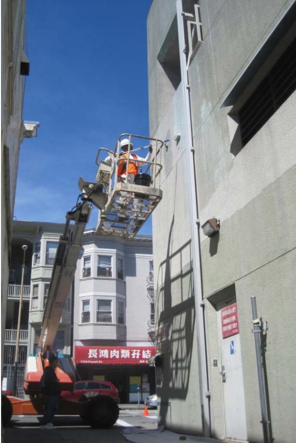
Station 2 Wall Primer Application
