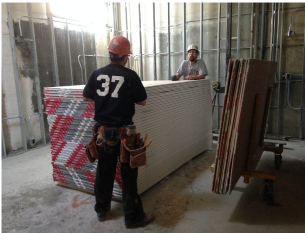
Crew Assembling Sheet Rock
