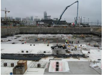
Construction activites at Basment level: mud-slab pour; protection slab installation; subgrade waterproofing; reinforcement at pile caps
