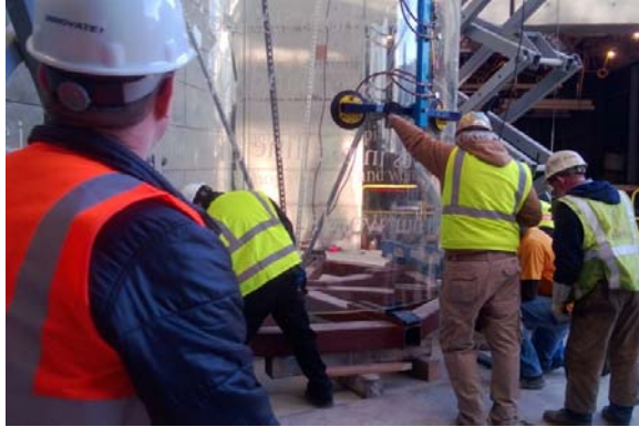
Installation of Police HQ Art
