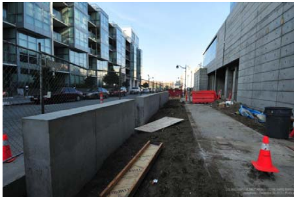
Anti-ram walls at China Basin St.
