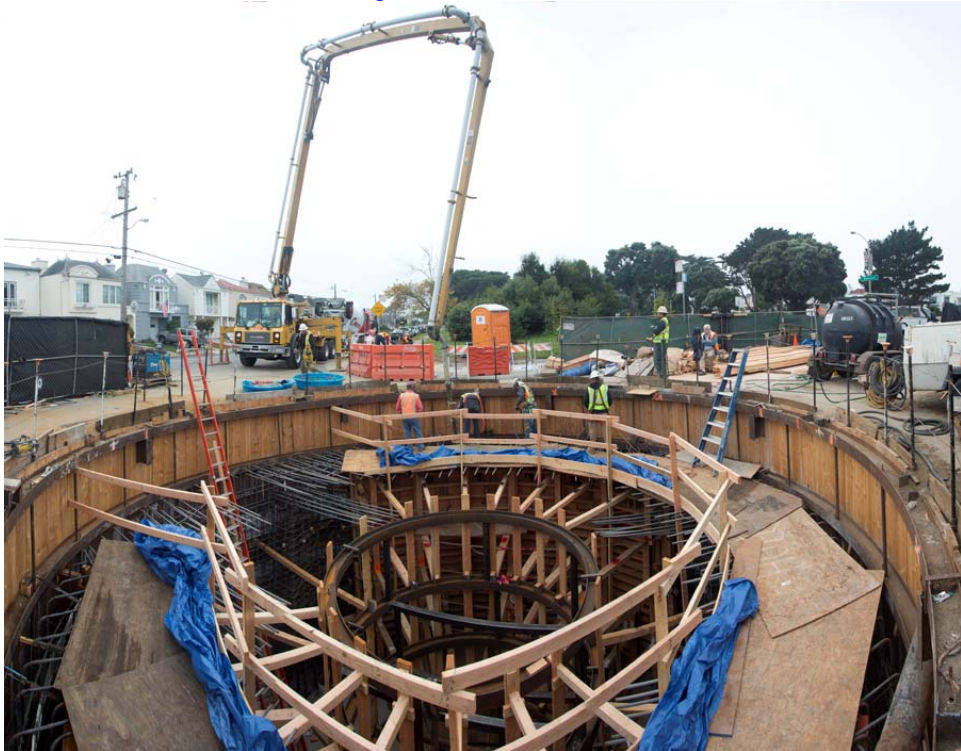
Placing cistern wall concrete
