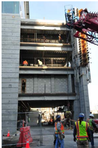
Conc. formwork removal
