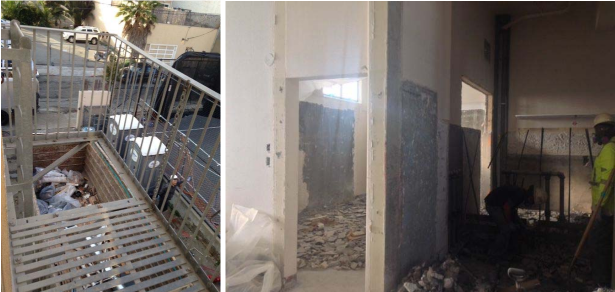
7427A Station 36 Selective Demolition
