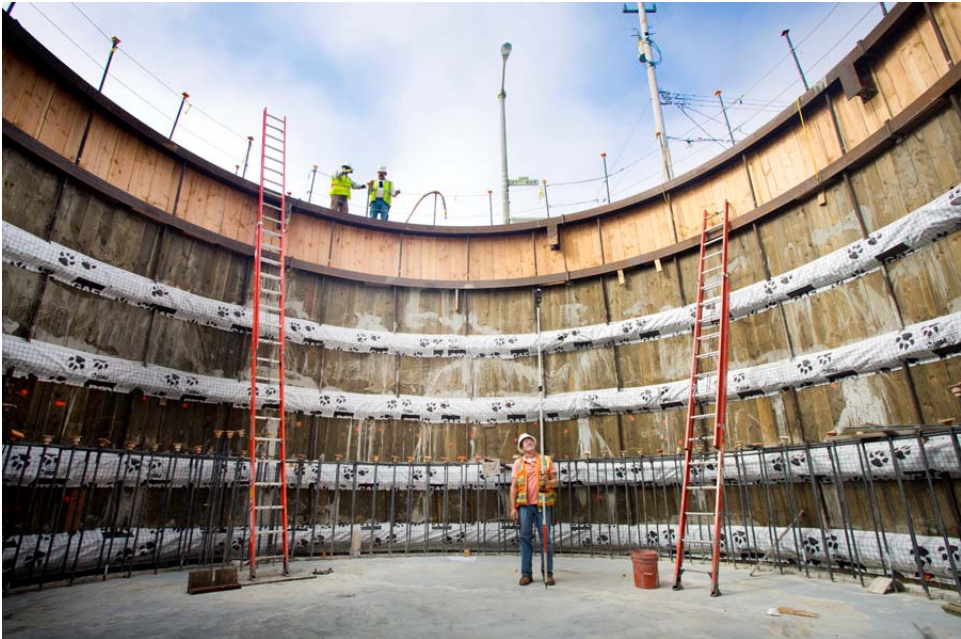
Confirming cistern floor slab elevation
