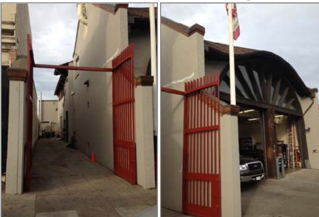
7436A Exterior Envelope Station 42
