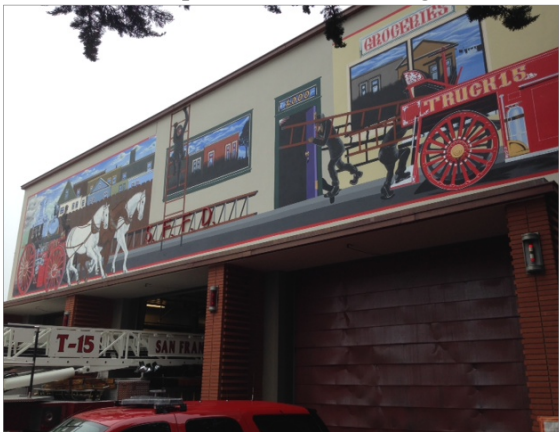
Exterior Envelope Station 15 Painting
