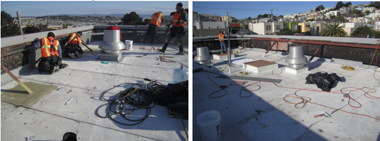
7438A Station 44 Roof Replacement
