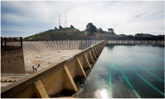
Twin Peaks Reservoir Joint Sealant
