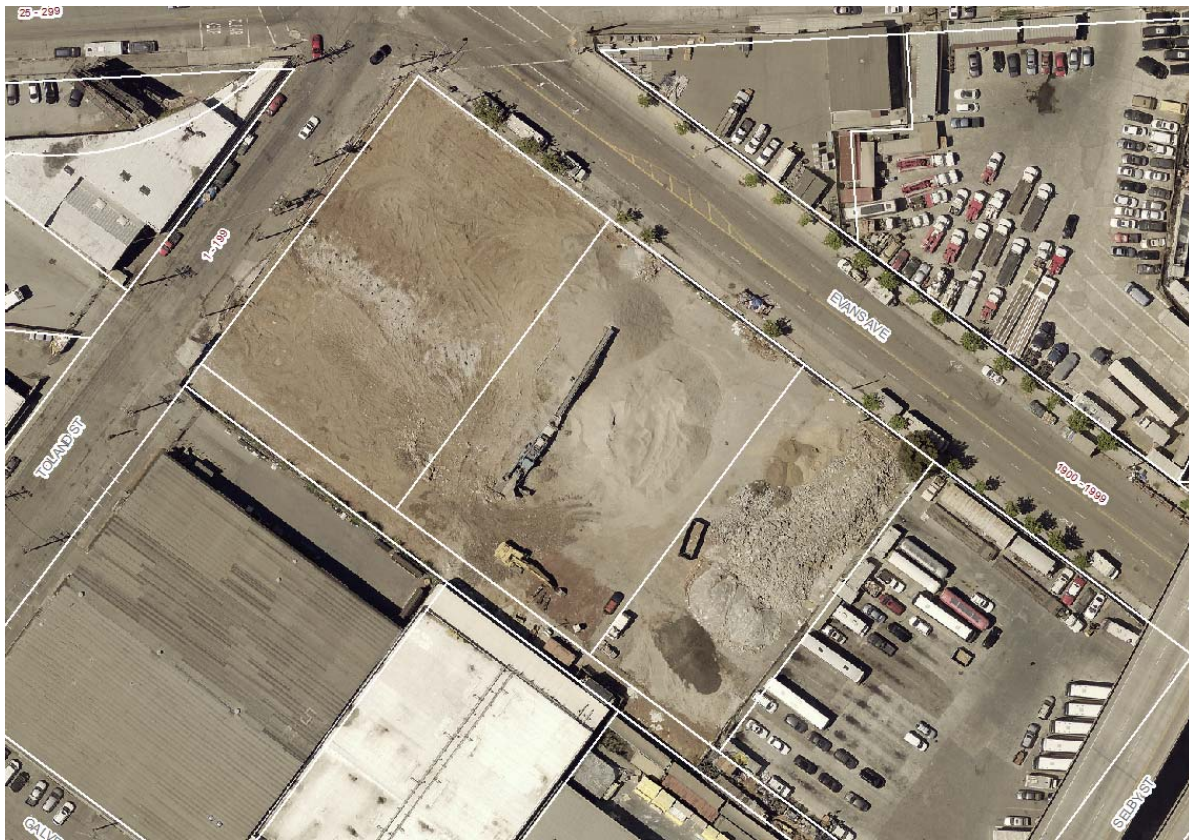
Aerial Photo of 1995 Evans Avenue Post-Demolition (2018)
