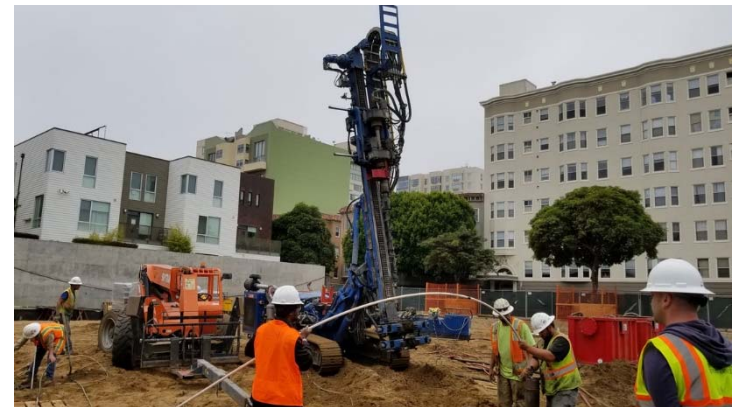
FS 5 Drilling and Placement of Soil Micropiles
