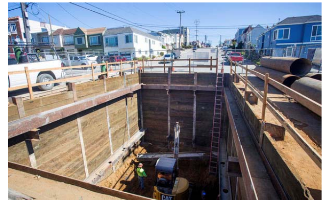
Cistern under construction
