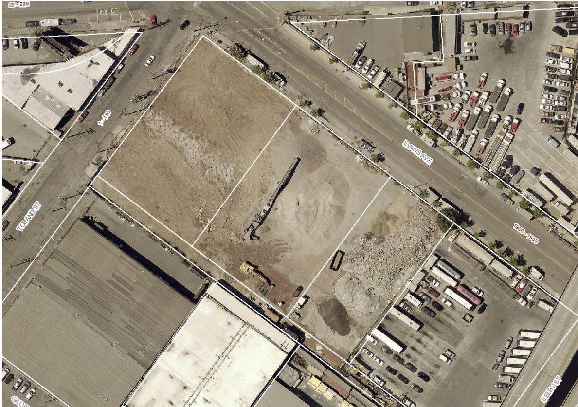
Aerial Photo of 1995 Evans Avenue Post-Demolition (2018)
