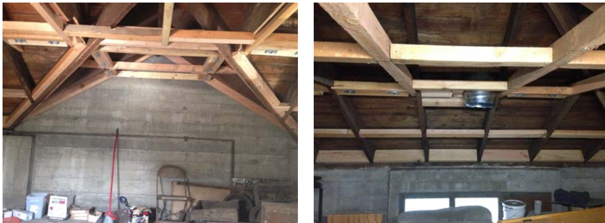
Structural work in attic
