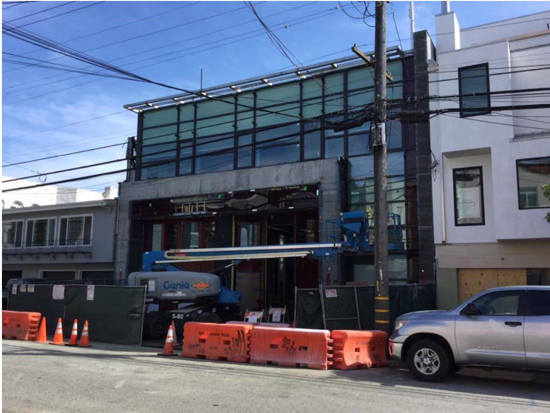
North Elevation on Greenwich Street (September 26, 2018)
