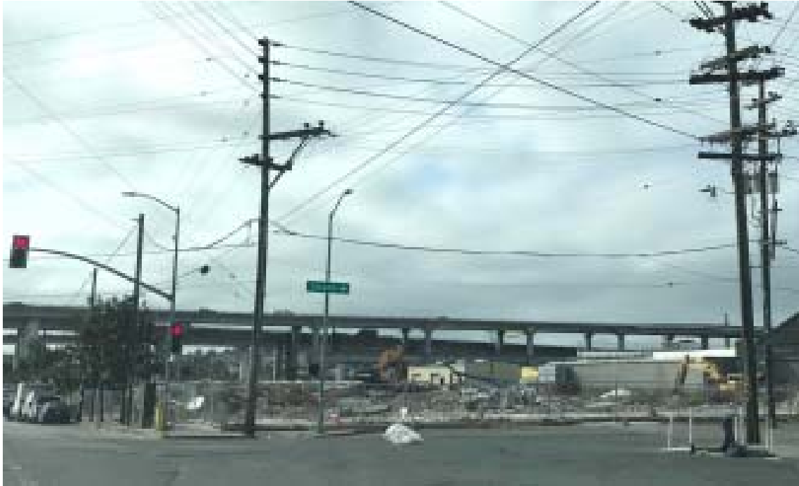
Demolition of Existing Bakery (July, 2018)
