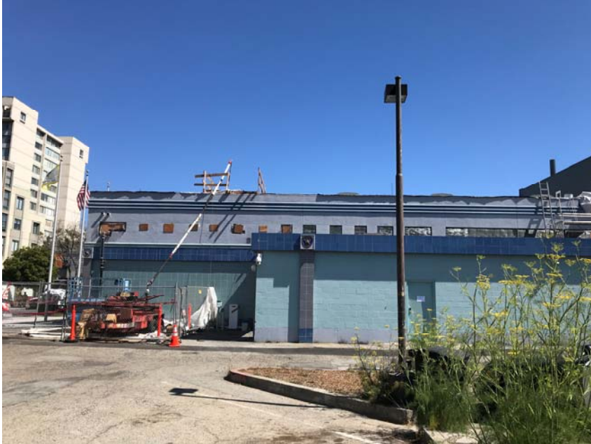
Structural strengthening and exterior stucco wall repair
