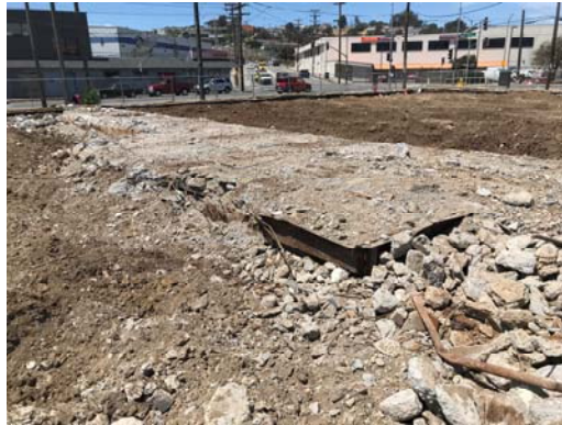
TCFSD – Existing Buildings Razed at 1995 Evans Ave.
