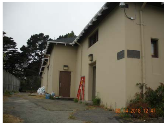
Hazmat abatement and paint stabilization on gutters to be demolished
