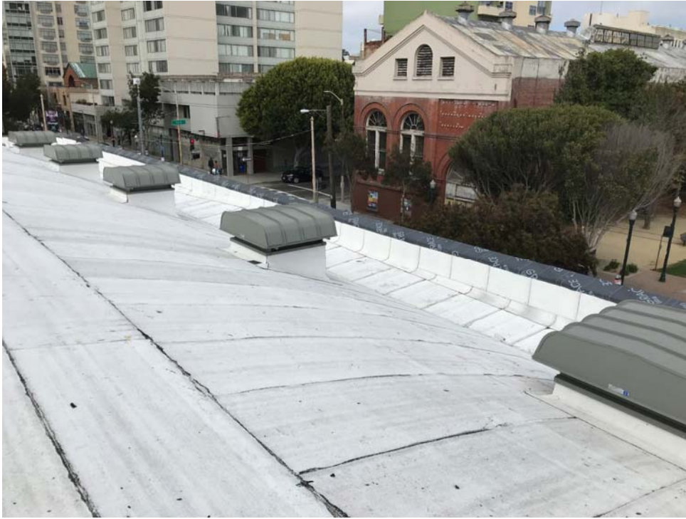
New roof vents
