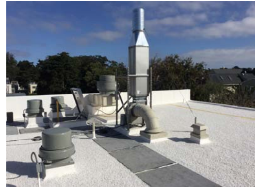
FS 22 Roof and Exterior Envelope – Complete
