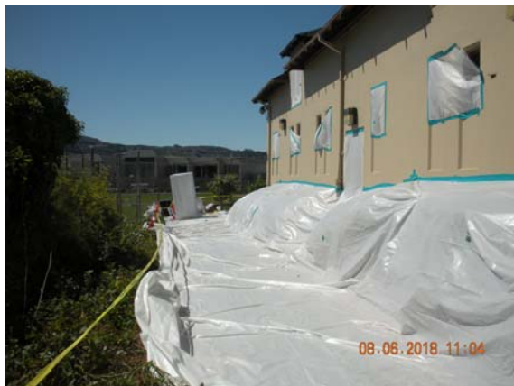
Hazmat abatement and paint stabilization on gutters to be demolished
