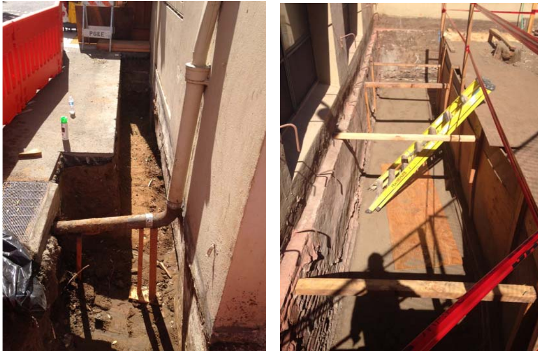
Excavation in preparation for new shotcrete wall and foundation
