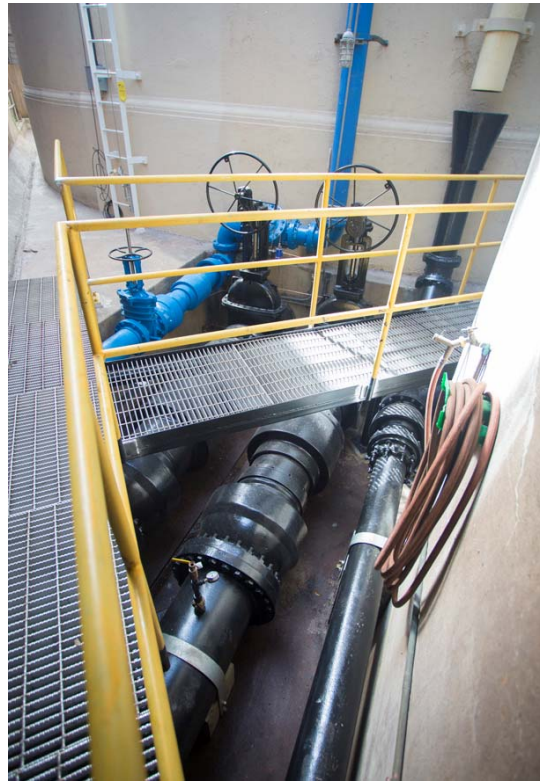
Jones Street Tank, new piping and walkway
