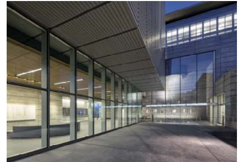
Photo © Tim Griffith, 2015 Entry courtyard
